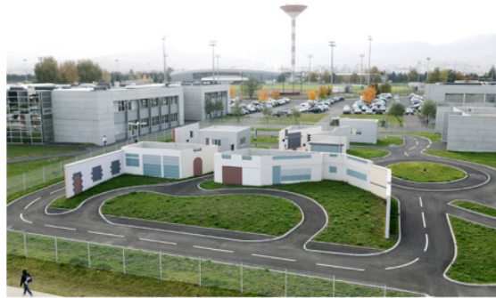
Figure 1.1: PAVIN test track in Clermont-Ferrand (France)
