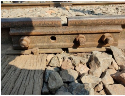
Fig. 4. Broken fishplate.
