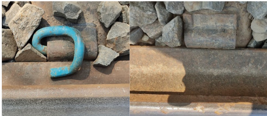
Fig. 2. Correct clip v broken clip.
