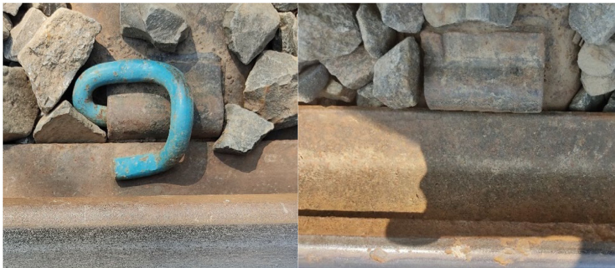
Fig. 2. Correct clip v broken clip.
