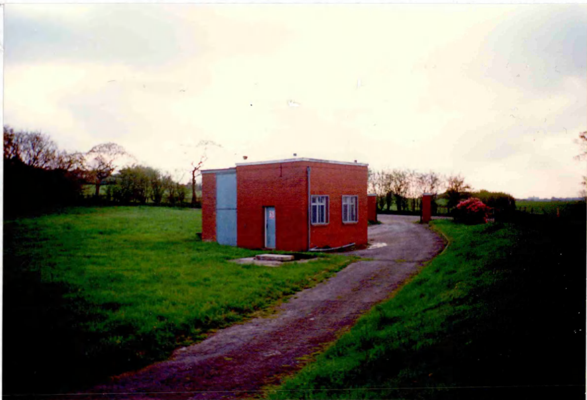
Figure 4.1. The pilot plant building at Lostock WTW.
