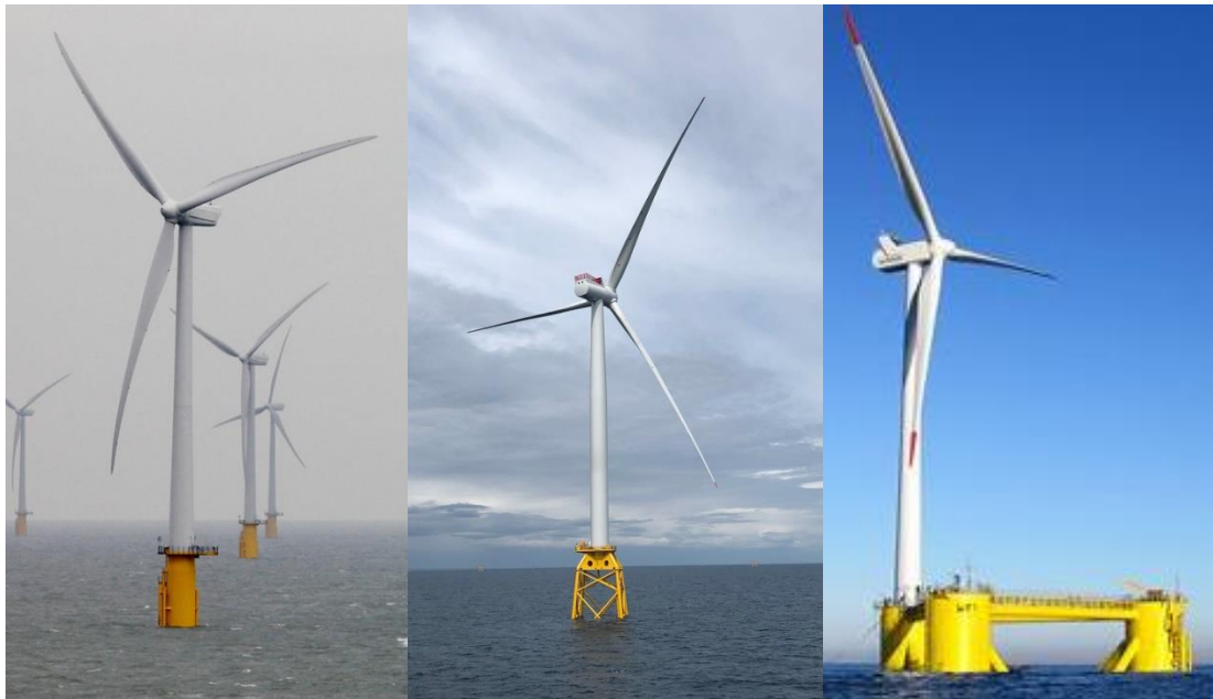
Figure 2 Thanet offshore wind farm 5 MW turbine (left) standing on a monopile foundation (image modified from Werdigier, 2010). Beatrice offshore wind farm 7 MW turbine (centre) standing on a jacket offshore wind farm (image modified from 4C Offshore, 2019). Wind float 2 MW test turbine (right) standing on a floating barge structure (image modified from Weyndling, 2019).
