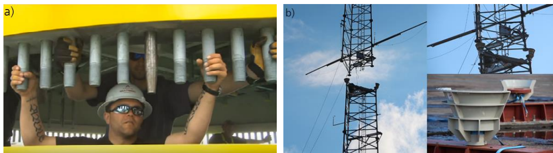
Figure 8. Current use of guiding systems: (a) Guide pins [30], (b) Guiding funnel [29].
