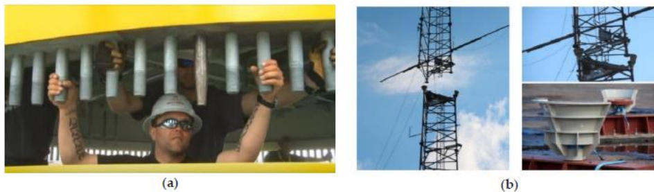
Figure 1. Examples of mechanical guidance systems: (a) Current use of guide pins; (b) Guide cones for human-free met mast installation [4].
