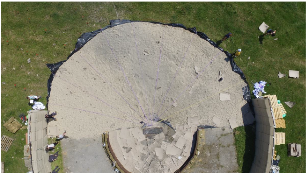
Figure 6. Aerial picture after detonation 1.
