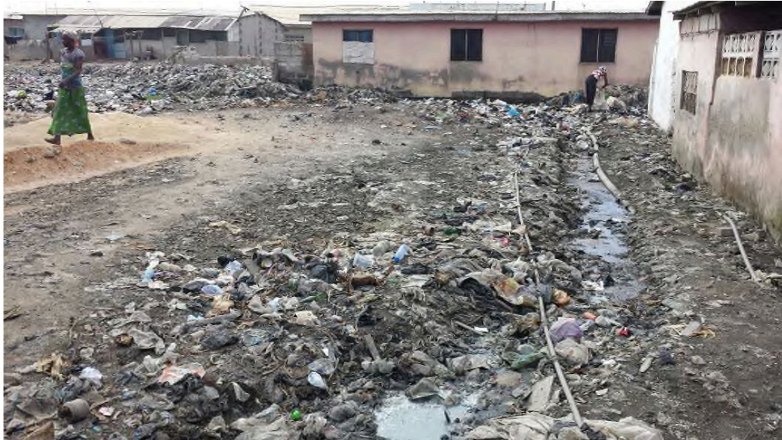
Figure 3: Watercourse filled up with rubbish and water marks on the houses
