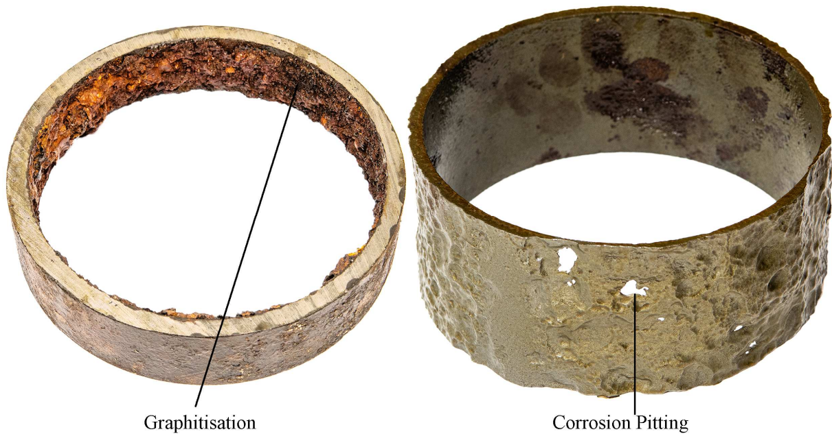
300 Figure 6. Cast iron pipe corrosion and chemical degradation.
