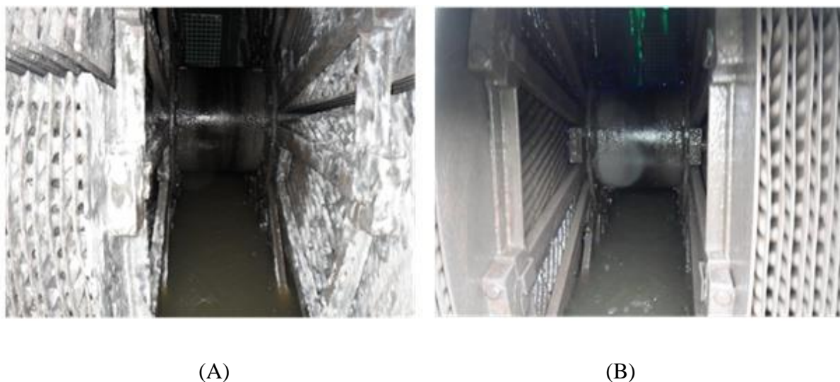
Figure 7. Image A shows the biofilm appearance on RBC 1 (1), image B shows the biofilm on RBC 2 (1).
