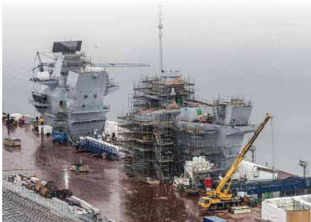
HMS Queen Elizabeth under construction (Crown Copyright 2014- Photographer-Andrew Linnett)
