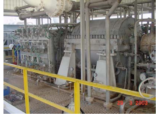
Figure 1—7 Horizontal split type. (PDO,Lakwair,2003)
