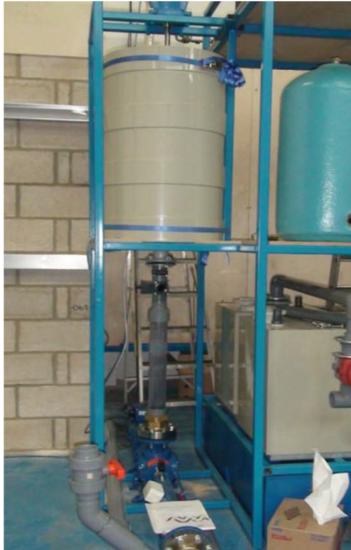
Figure 3-3: Slurry mixer and pumping system
