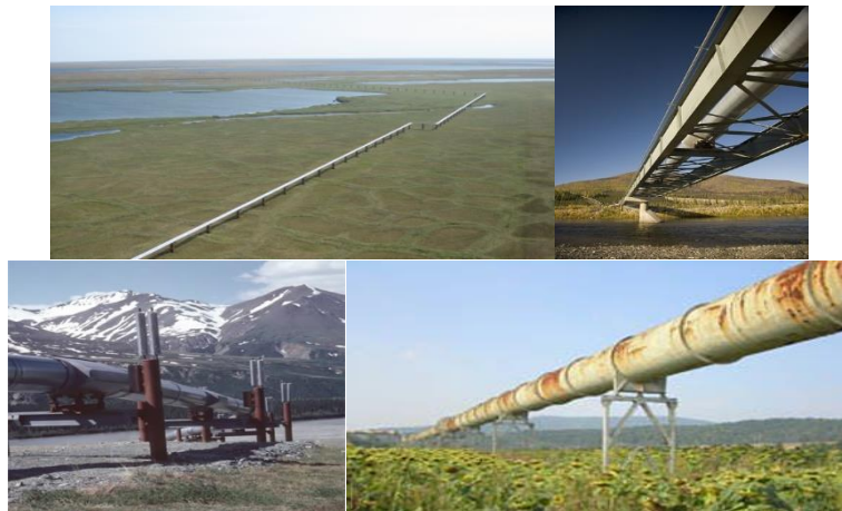
Figure 3-26: Pipeline structures samples, Ref: Image collection was produced from reference (Oil & Gas Pipeline, 2011)
