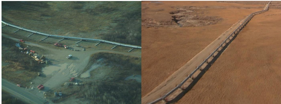
Figure 4-1: Two images of a pipeline at various environments (Pipeline Surveillance Company - Not for Public Release, 2012)
