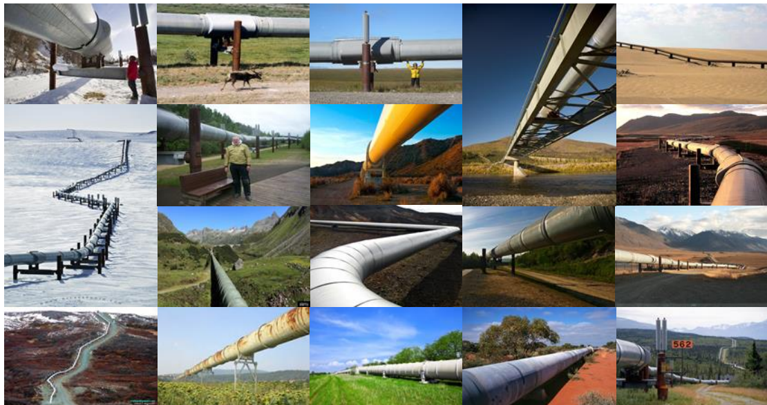
Figure 2-5: Environments of pipeline infrastructure, Ref: Image collection was produced from reference (Oil & Gas Pipeline, 2011)
