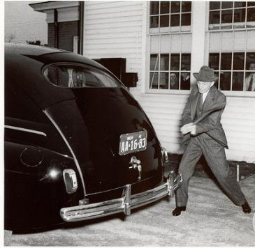
Figure 2-1: Henry Ford testing with an axe soy-bean based plastics [7]
