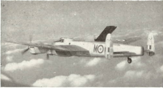
FIGURE 31. Lancaster with Midge wing on mid-upper fuselage.
