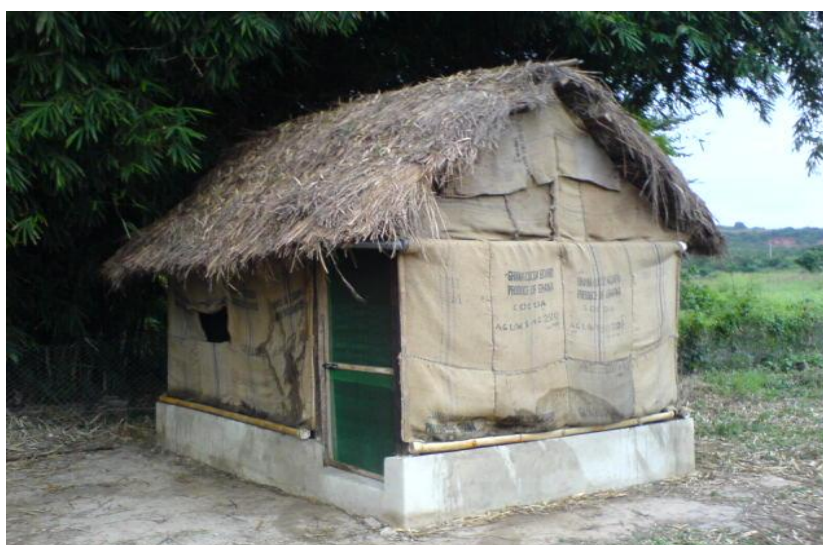
Figure 2.10 Evaporative cooling barn for sweetpotato storage in Ghana
