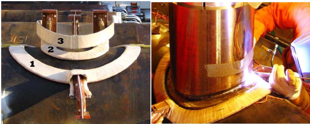
Figure 2-41: Three induction coils on a test pipe (left) and welding the branch (right) 39
