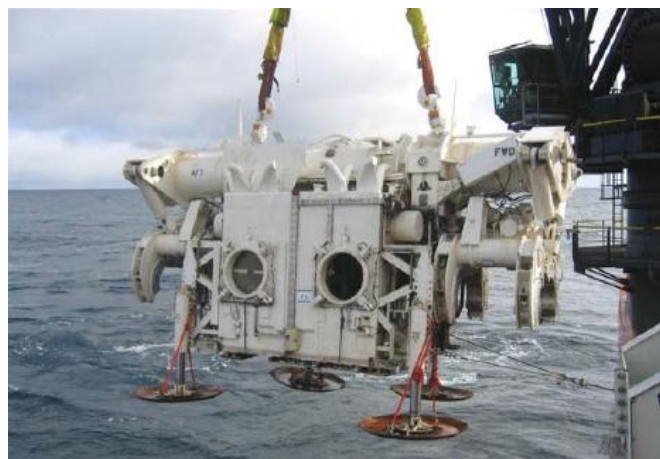
Figure 2-19: PRS welding habitat during installation for welding at Langeled pipeline 43
