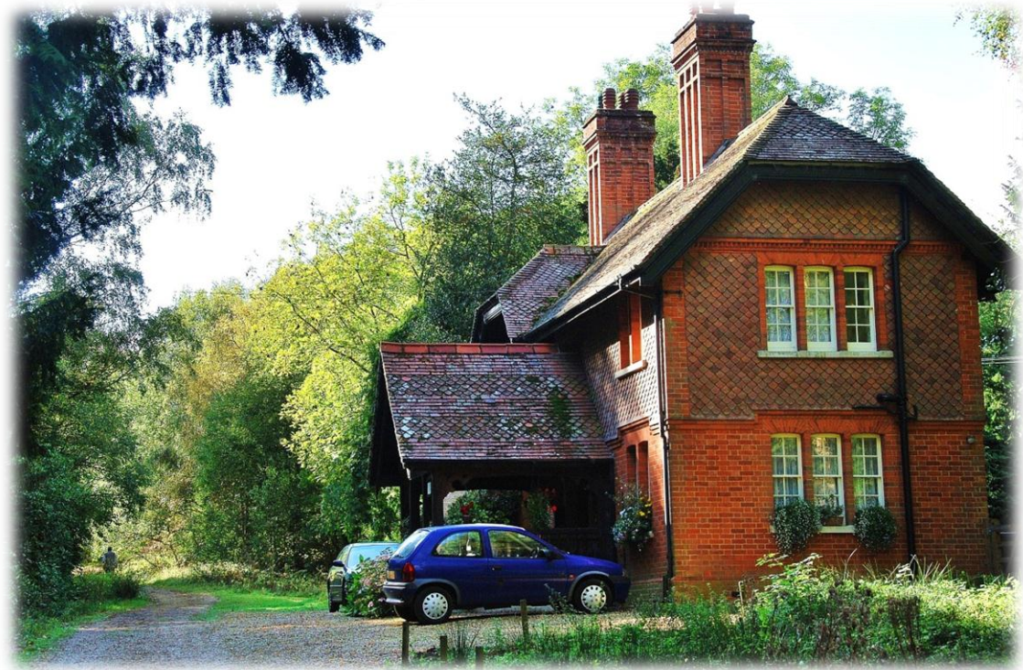
Plate 7:4: Fuller's Earth Lodge (vernacular building), New Wavendon Heath
