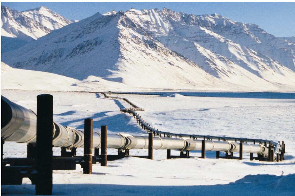
Figure 8.3: Snapshot of the Trans-Alaska pipeline (Smith, 1996)
