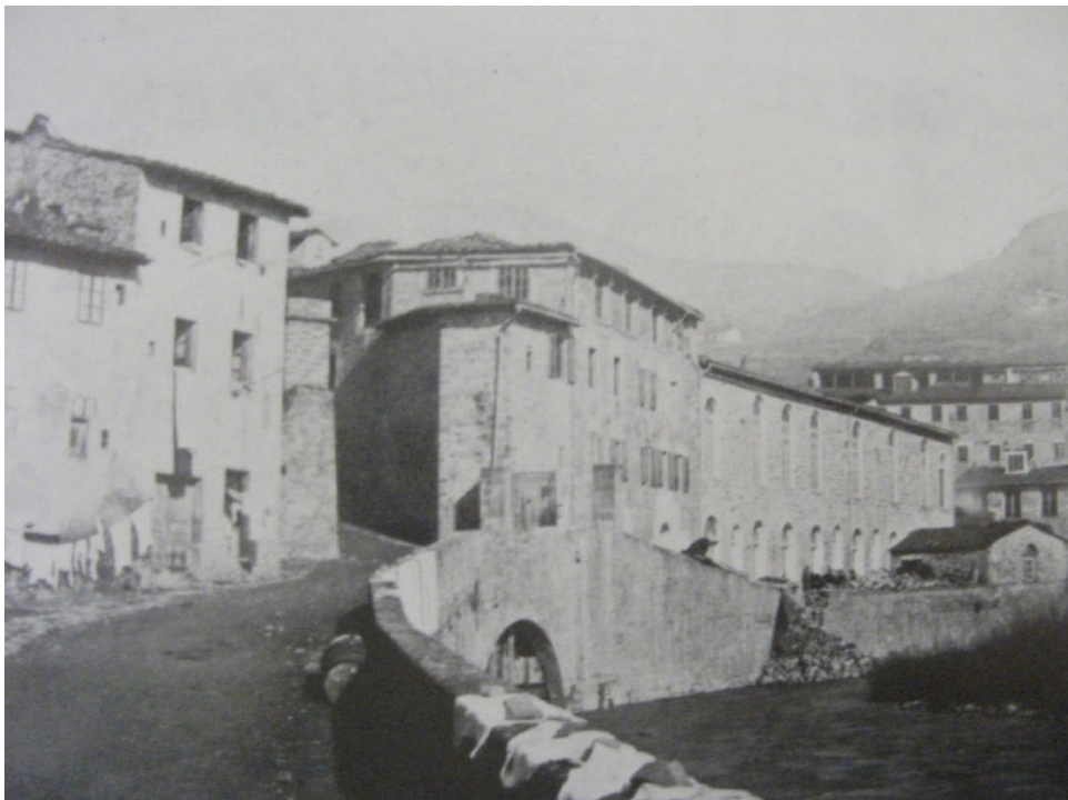
Figure 1 Lanificio 1930. Textile factory by the Arno affluent Staggia. Stia (AR) Italy (Della Bordella, 1998)
