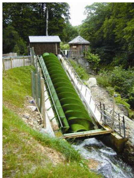
Figure 29 Archimedean screw turbine (co2sense.org.uk)
