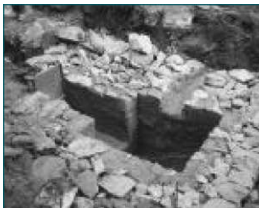
Figure 50 Forebay under construction (Singh and Ranjitkar, 2000)
