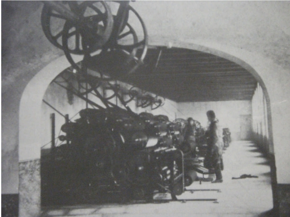
Figure 2 Mechanical hydropower to drive textile machines (Della Bordella, 1998)
