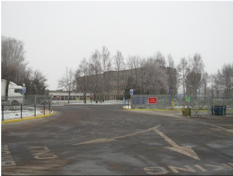
Figure 2.11: Entrance to Flixborough composting plant, showing proximity to sensitive receptors
