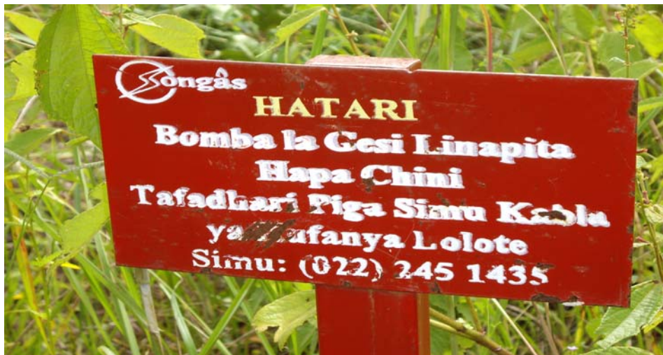
Photo 5.4: One of the signposts by SONGAS project at M'baya displaying a warning message that “DANGER the gas pipeline passes underneath”
