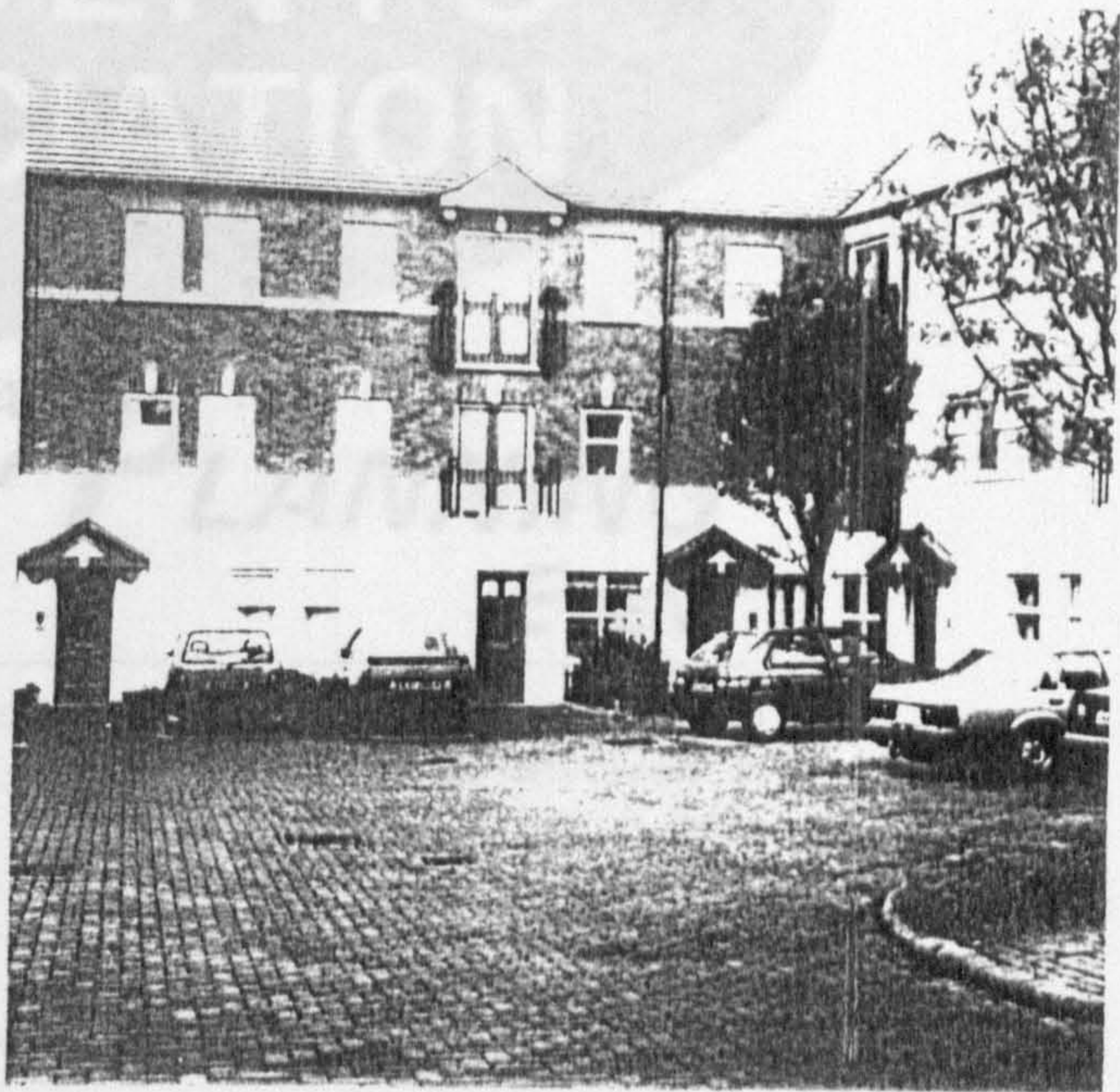
Shared Surface pedestrian priority surface direct access from property
