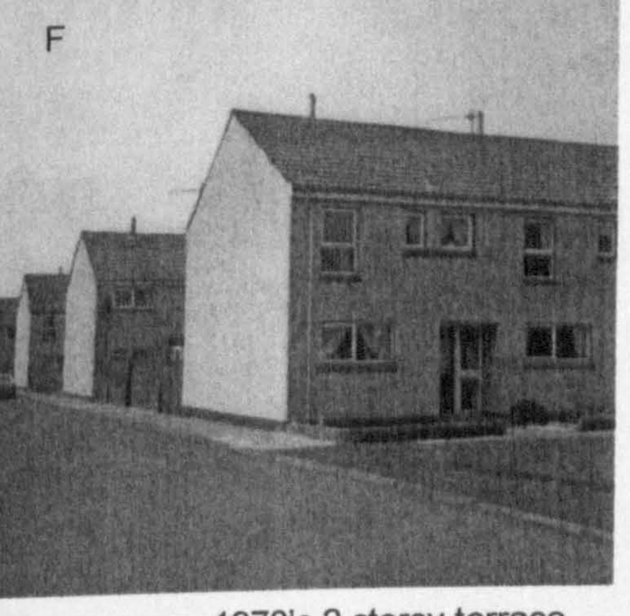
1970's 2 storey terrace (15-20 dwellings per acre)
