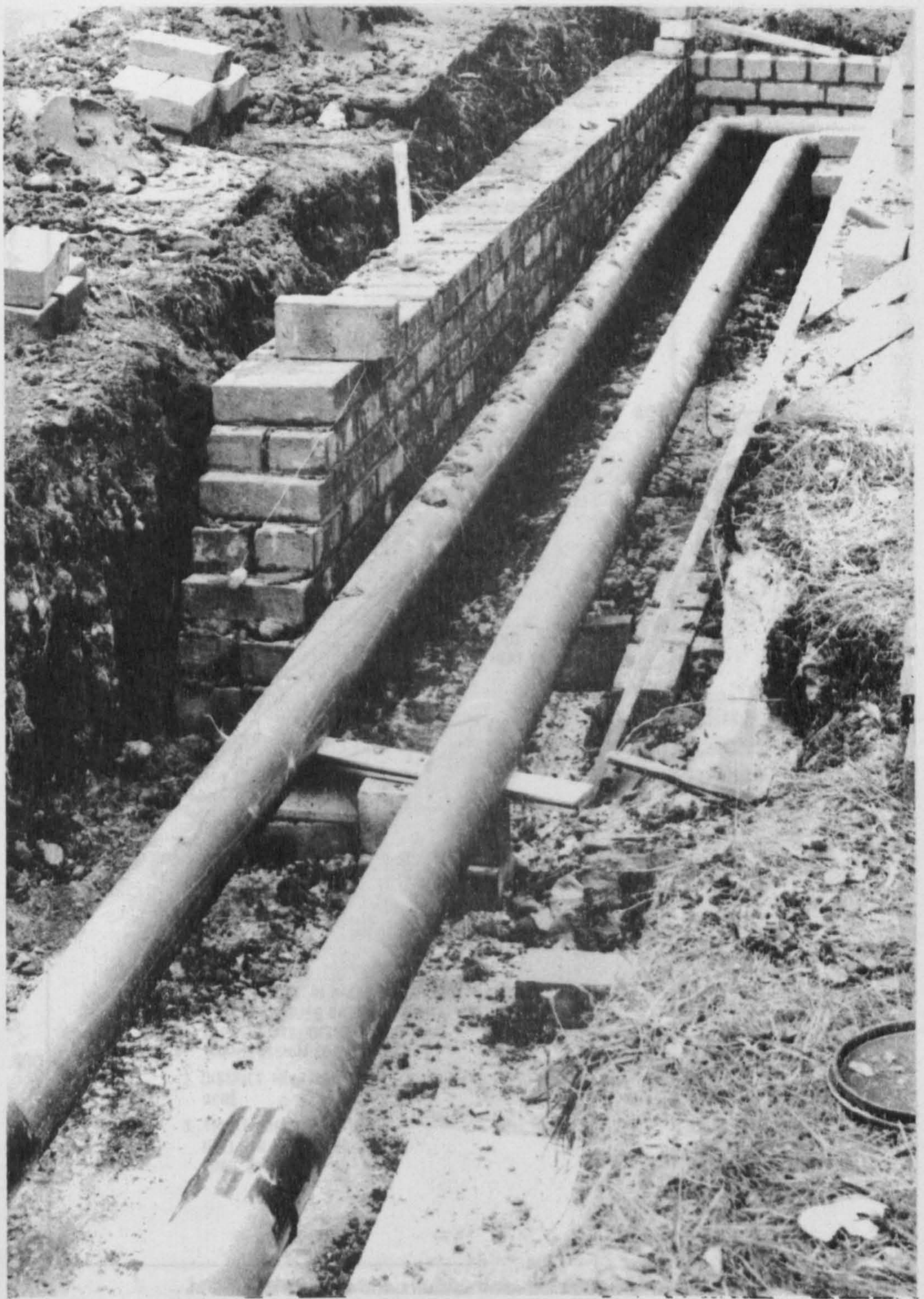
Fig. 1.10. Recent conventional practice, i.e. the 'side-by-side' arrangement of the 'outward' and 'return' district-heating pipelines in an air-filled rectangular trench.
