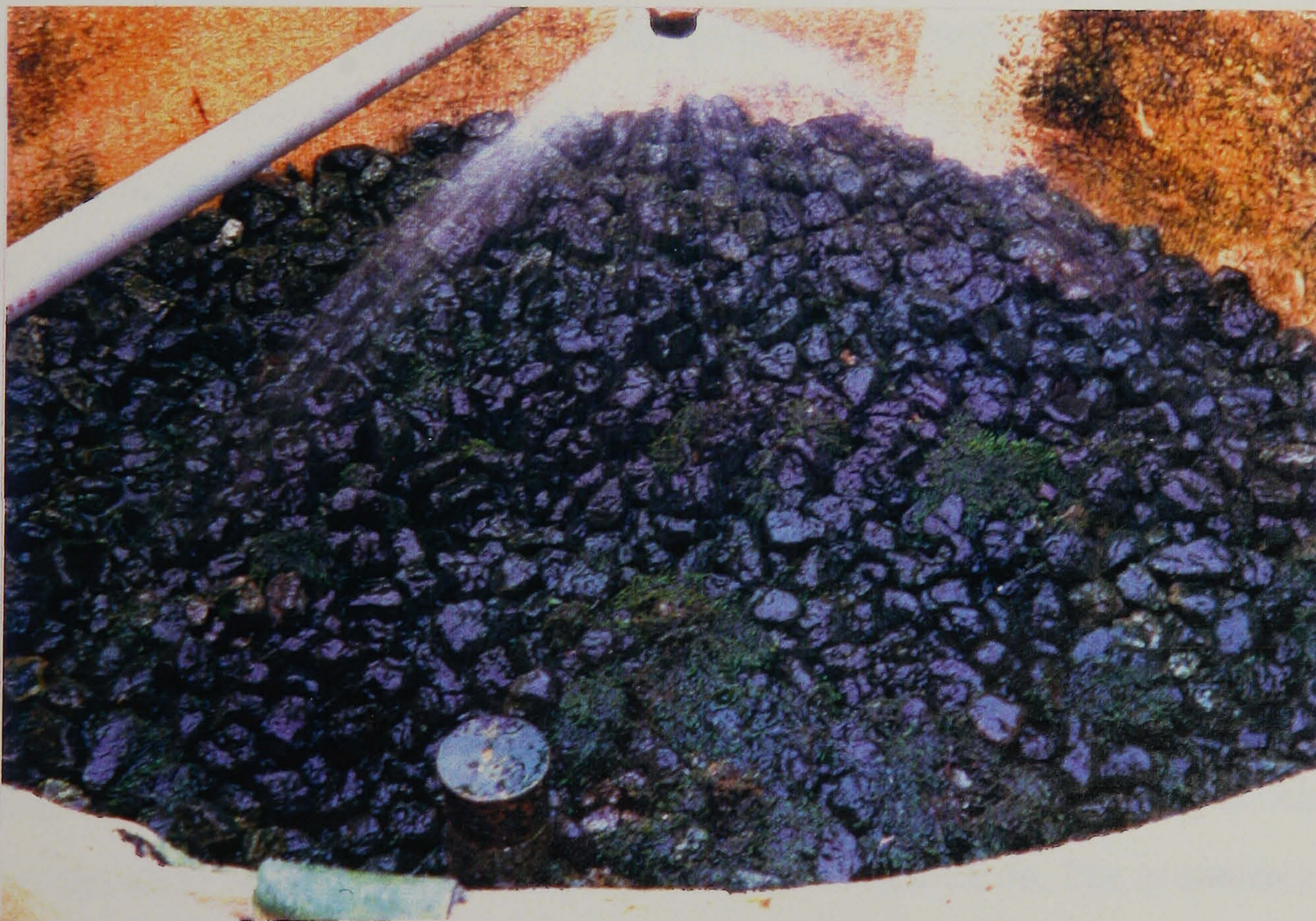
Plate 3: Effluent distribution in the blast furnace slag filter
