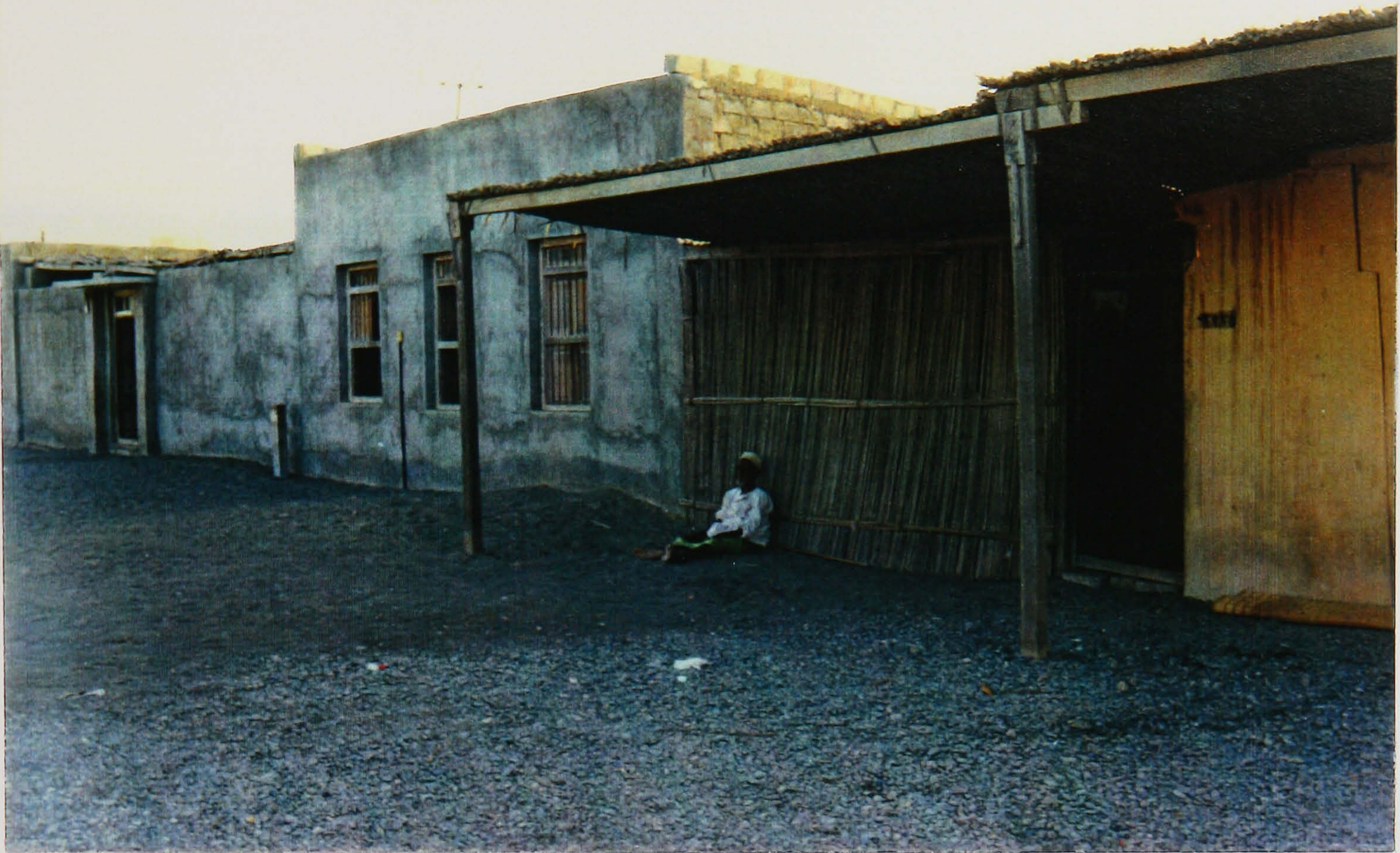
Figure 2.3(a): The use of palm-frond panels and shading-devices on the sea-facing wall of a vernacular house in Sohar .
