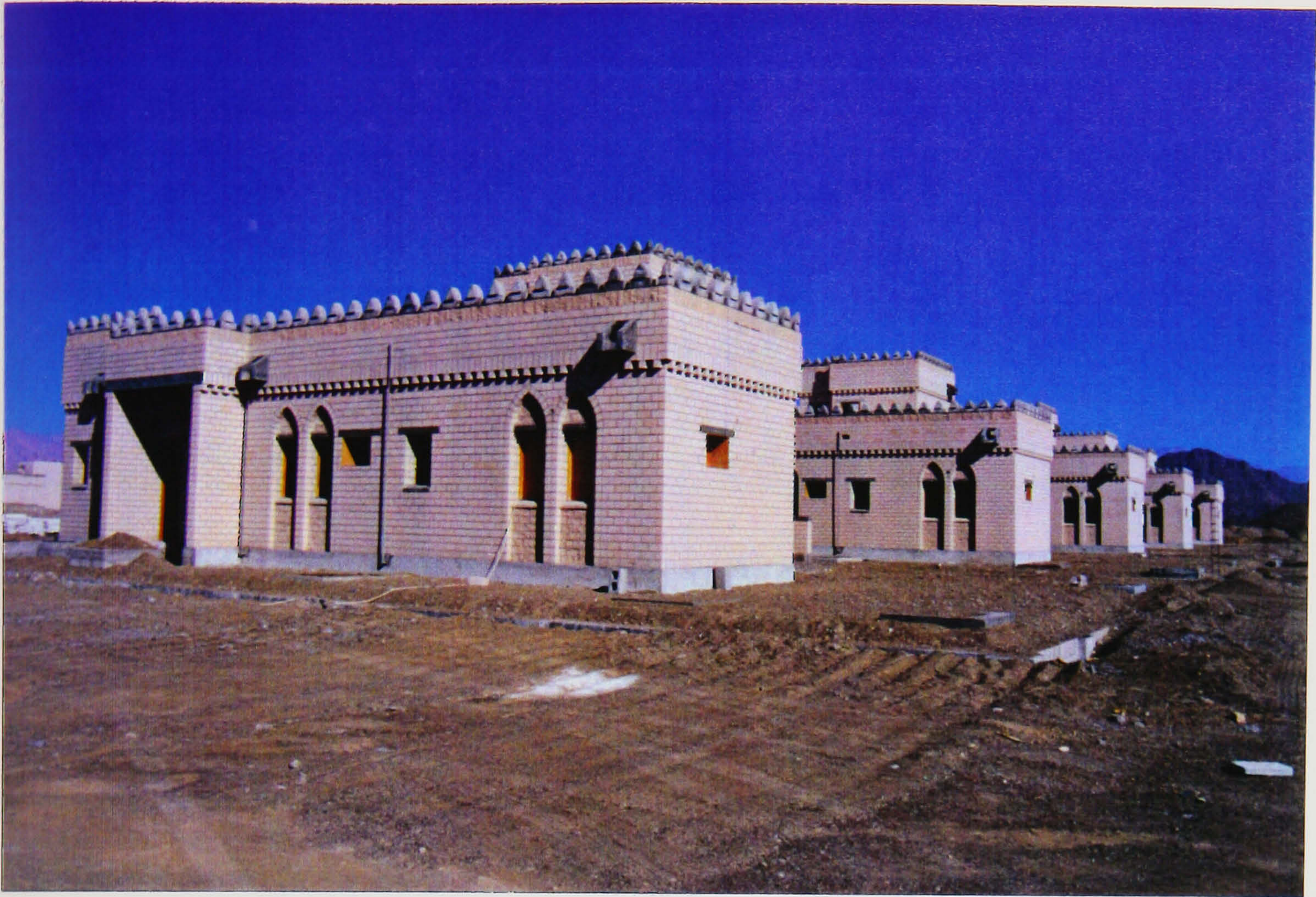
Figure 7.5: The house used to validate the single-room model, with insulated roof and un-insulated cavity brick walls.
