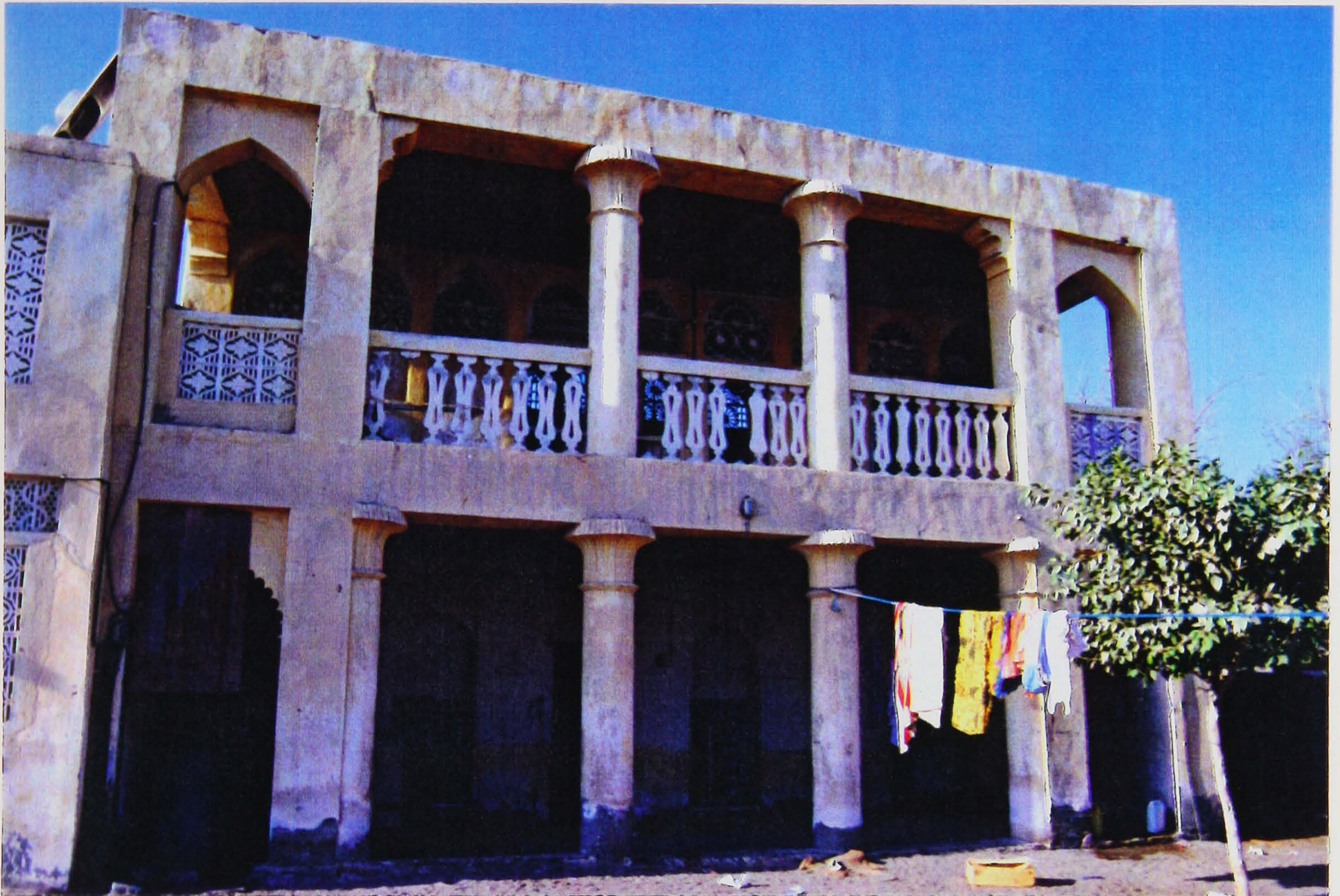
Figure 2.3(e): A vernacular house in Sohar . The house is designed to encourage air-movement and reduce solar gains, while maintaining privacy and security.
