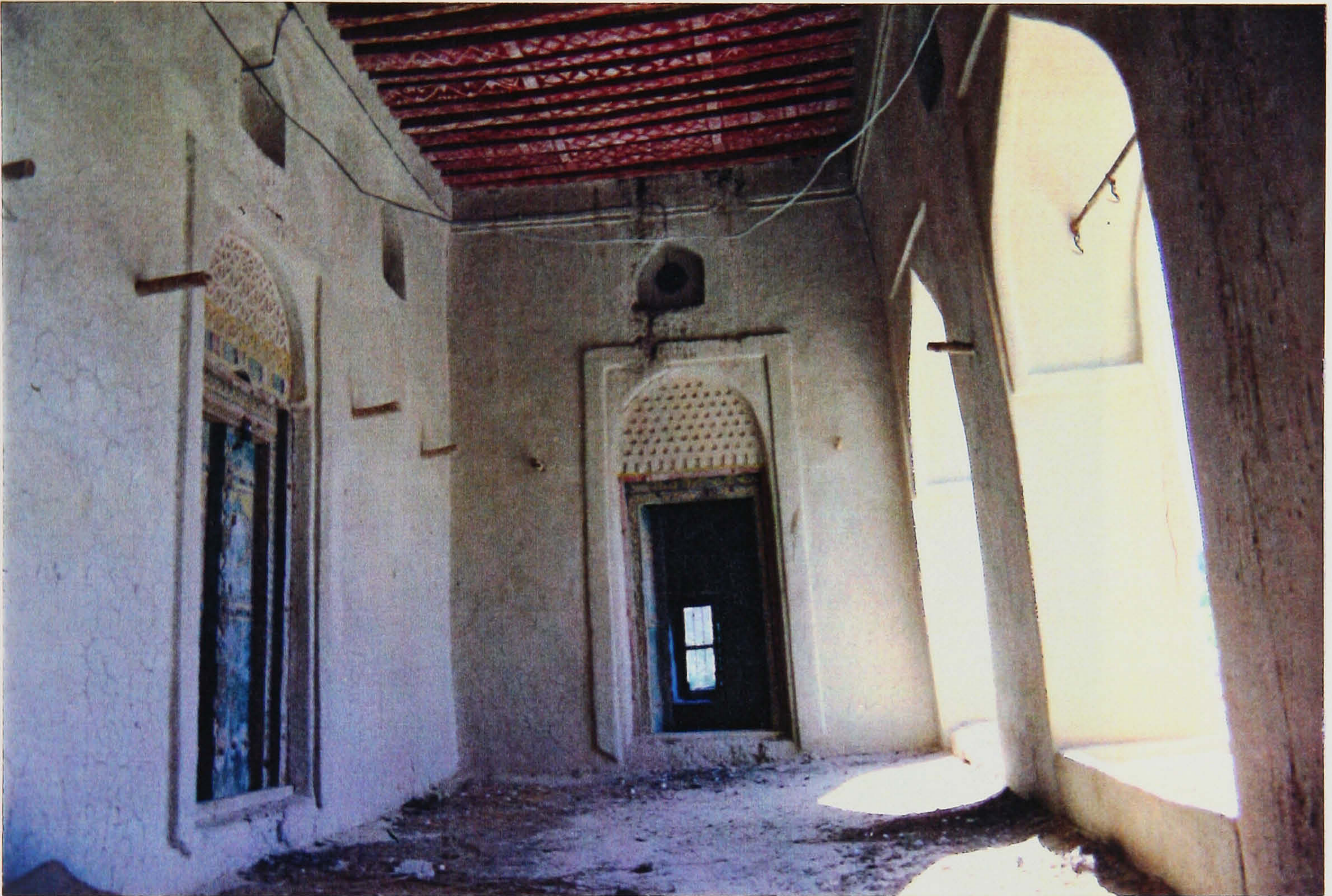
Figure 2.7(b): The inside of the "Dahreez" in the first story of the building in 2.7(a).
