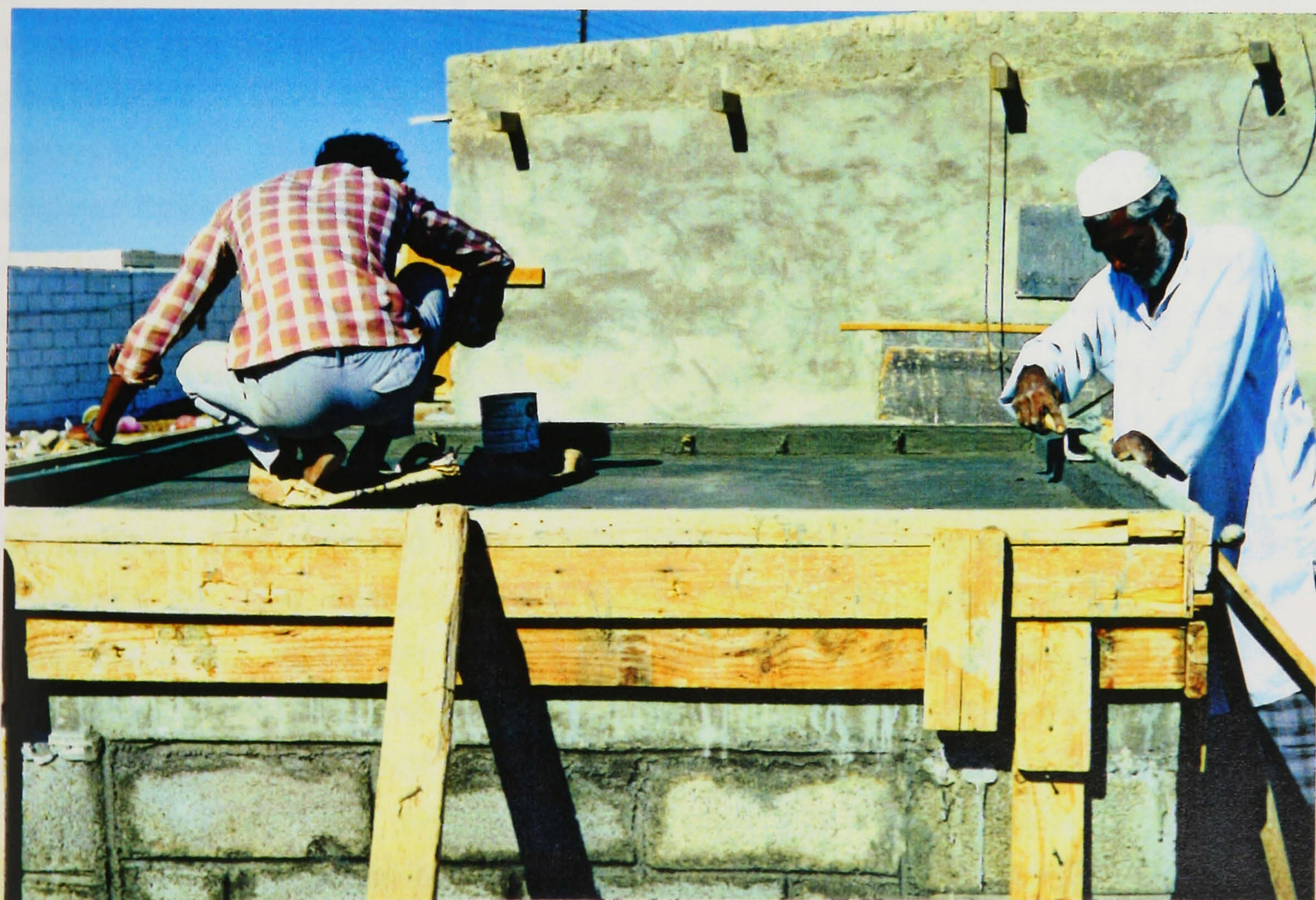
Figure 7.16: The Water Diode roof pond under construction.
