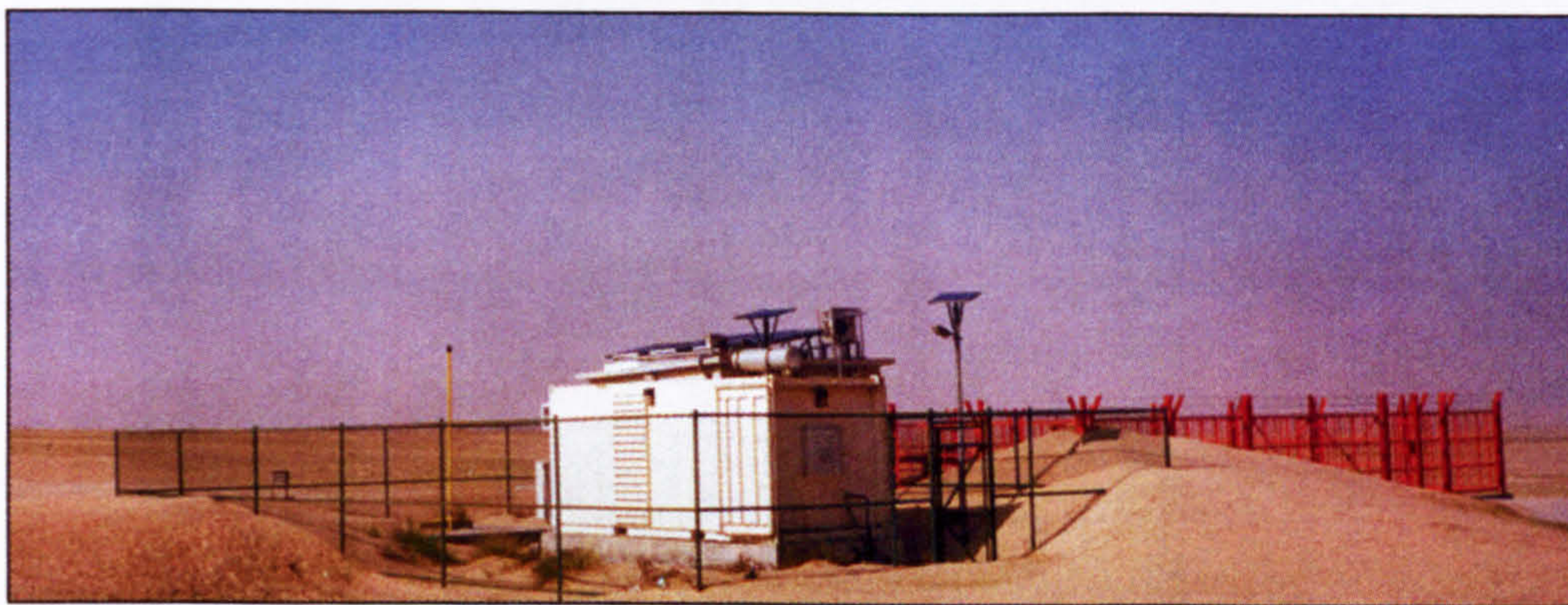
Figure 1.1: Sand drift at electricity transformation point in the desert of the State of Kuwait. Photograph by author in December 1999.
