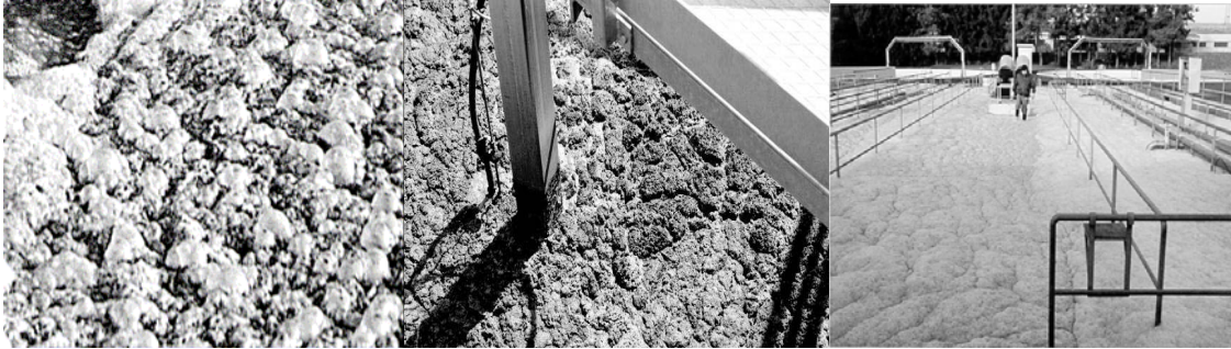
Figure 2.2: Foam covering an activated sludge plant
