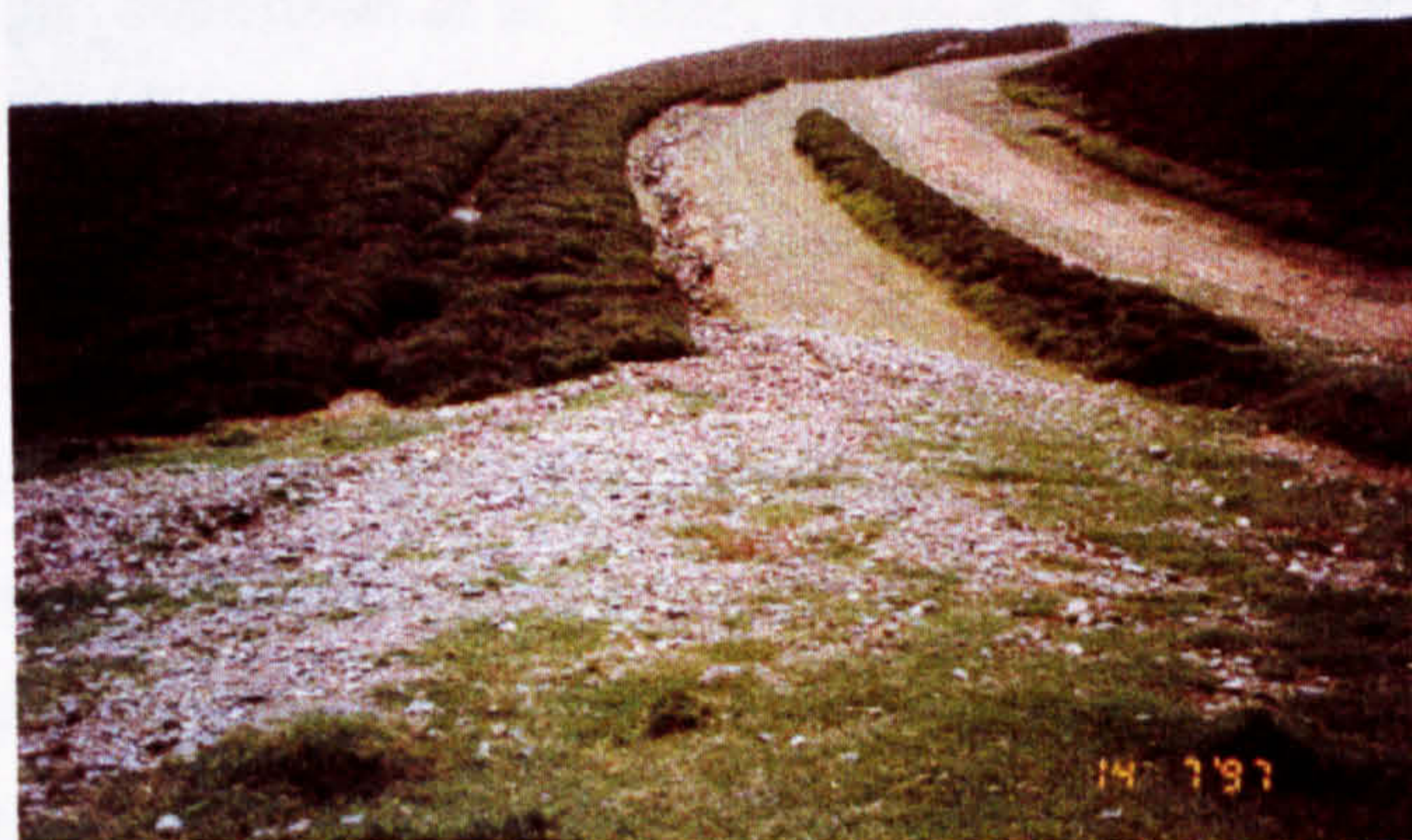
Plate 2.5 As well as detracting from the landscape, tracks across moorland are important runoff channels and sources of sediment (Quantocks, Somerset).
