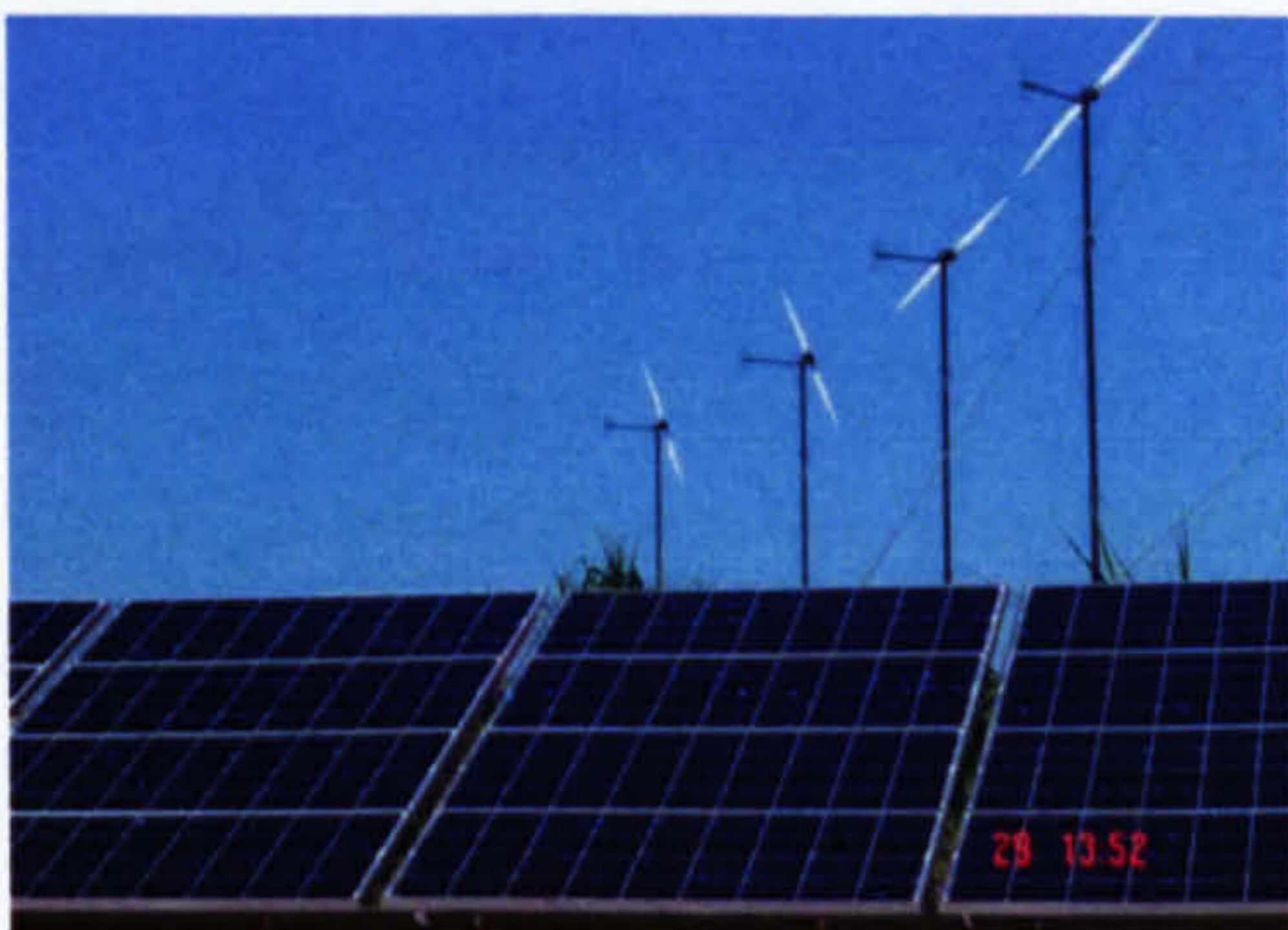
(a) 10 kW e wind-solar hybrid power system in St. Martin Island
