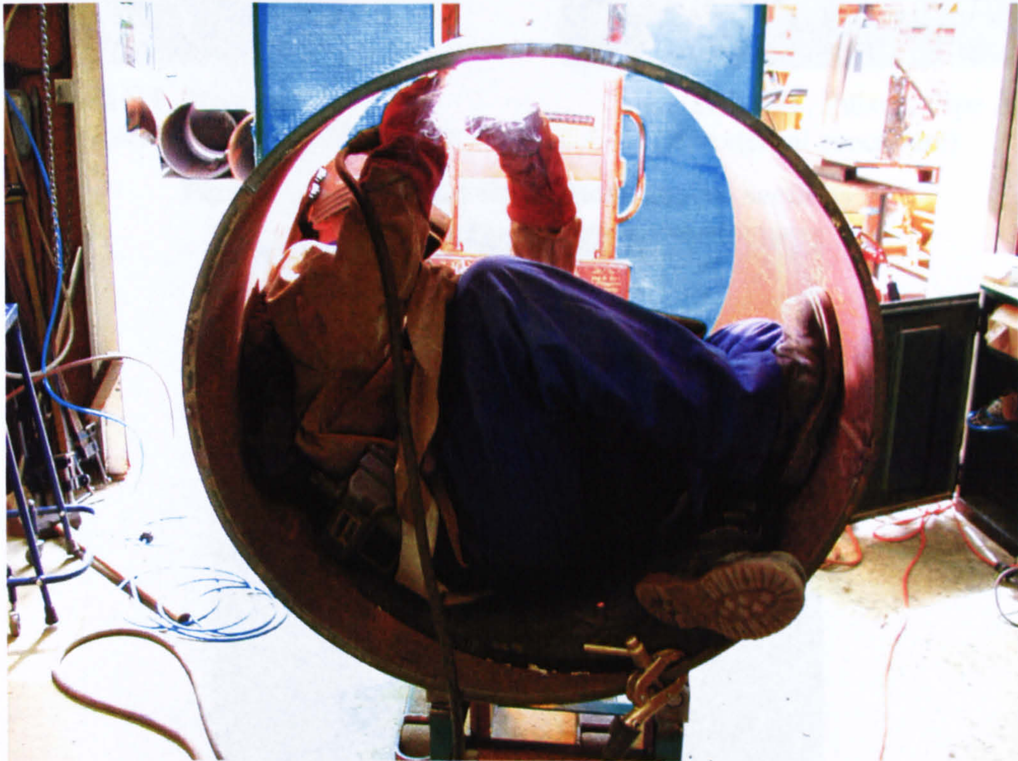
Figure 5-14: Typical repair procedure welding (internal root repair)
