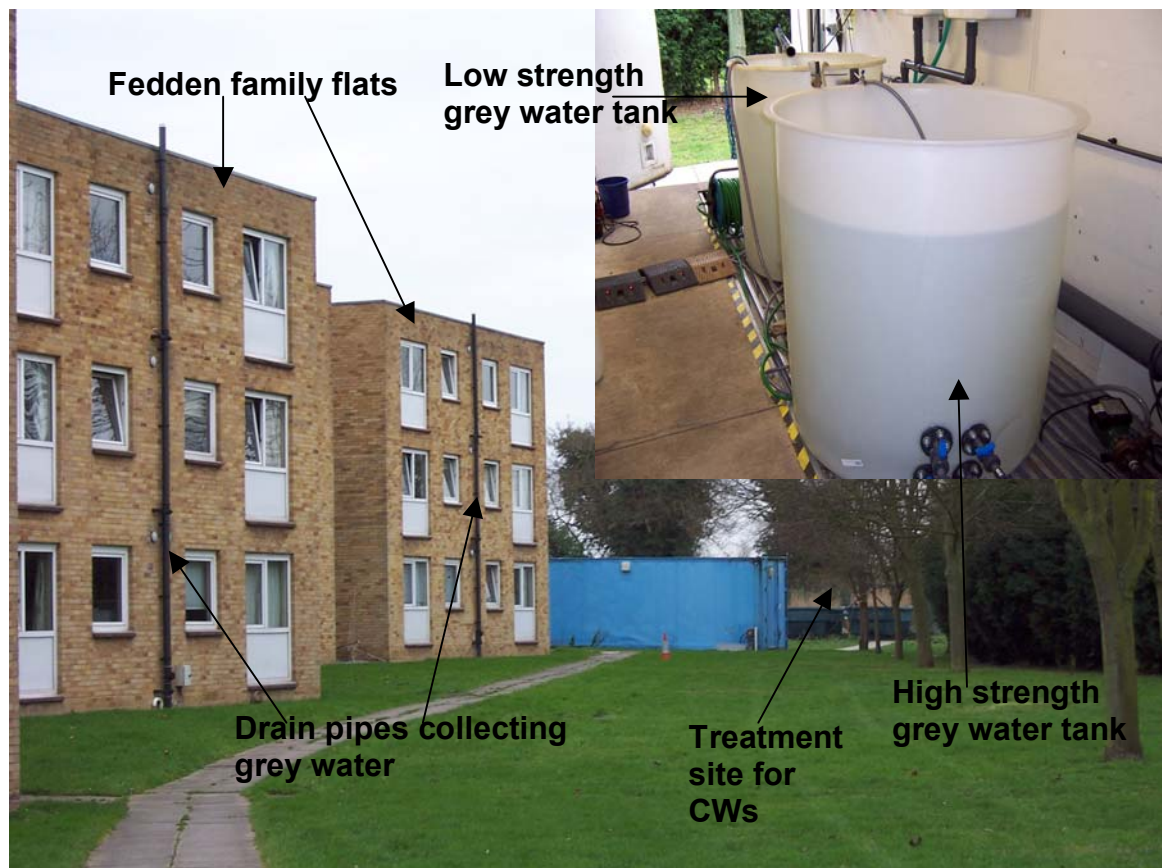
Figure 3.1.1: Grey water collection system showing Fedden family flats, pipe network which channels grey water to holding tanks in container (inset) and study site.
