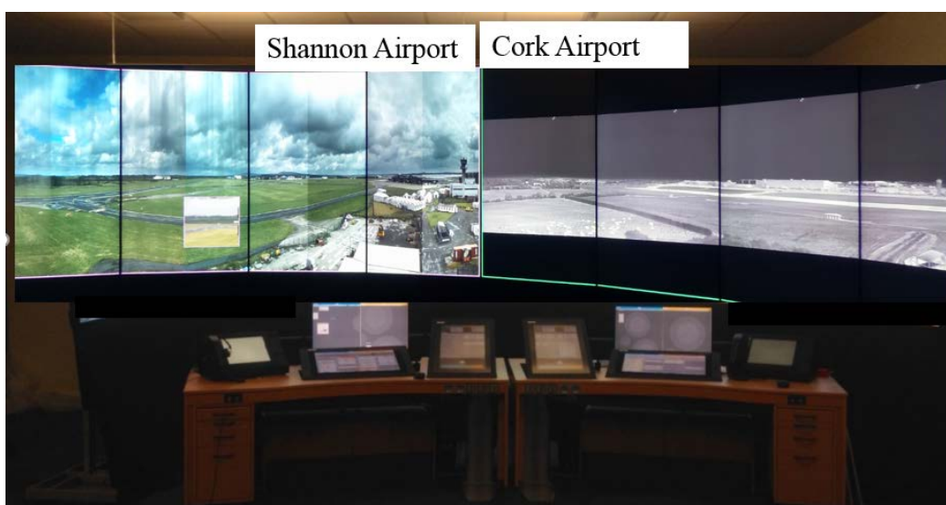
Figure 6.1. The Remote Tower Centre located at Dublin Airport in excess of 100 miles away provided air traffic services for both Cork and Shannon airports
