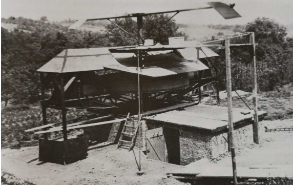
(a) Early test rig developed by Albert Hirth in 1914 (reproduced from Gersdorff and Knobling [7])
