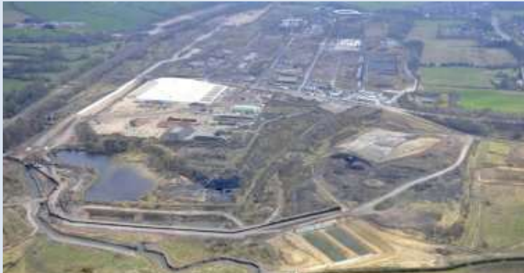
Aerial view of the site – during remediation
