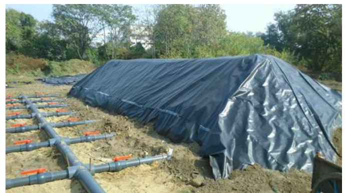
Figure 2.3. Soil Pile Design
