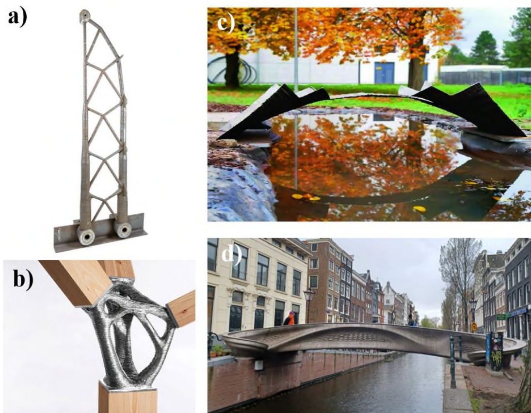
Figure 1: Successful examples illustrating the potential of WAAM in steel construction. a) Truss structure with optimised member sizes [16]; b) connection of spatial shells [17]; c) the bridge in Darmstadt [18]; d) MX3D bridge in Amsterdam (Photo taken by the authors). Reprinting permission for these images has been obtained from the publishers[16]–[18].
