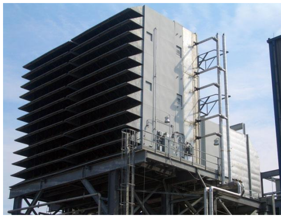
Figure 4-2 Intake filtration weather hood (Source: Pneumafil, 2016)
