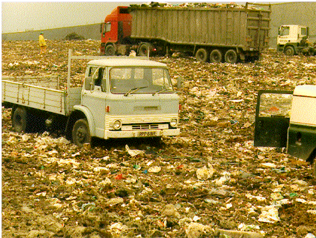
Figure 1.1 Lorries depositing waste at the tipping face of a MSW landfill site.
