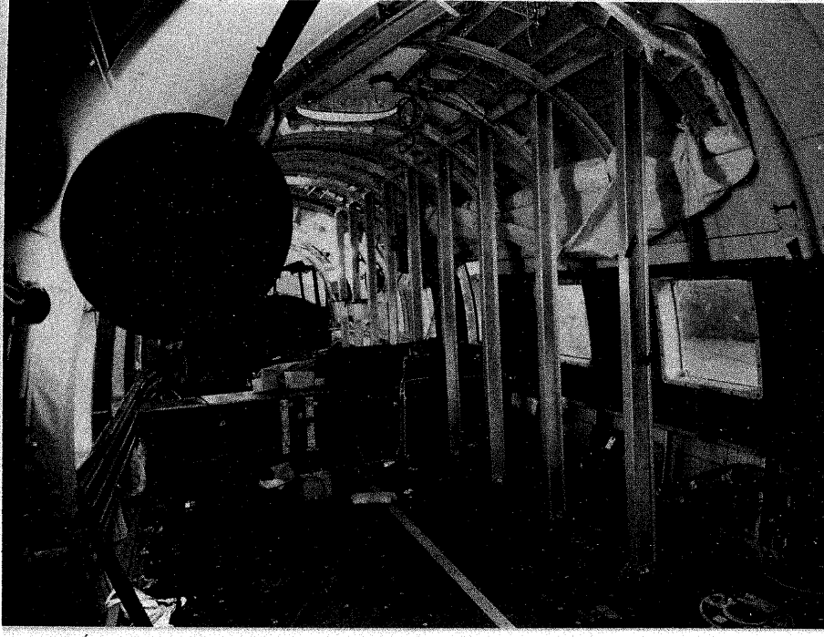
FIG. 11. INSTALLATION OF STANCHIONS FOR SPECIAL RACKING - IN PROGRESS VIEW LOOKING FORWARD
