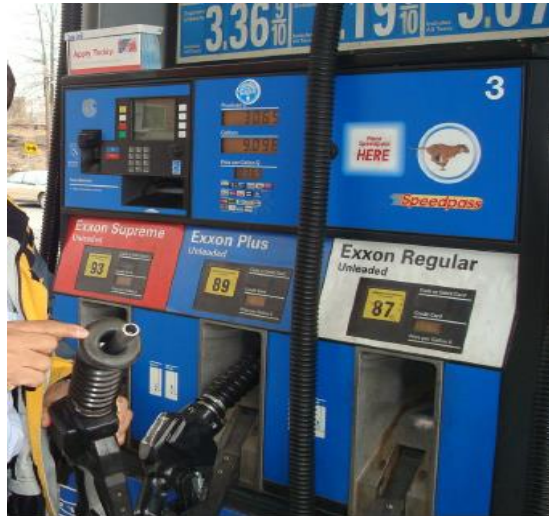
Figure 2-14: Balance-Type Stage II Nozzle of Gasoline Vapour Recovery Systems (Photo by Ahmed Alyami, 2008).
